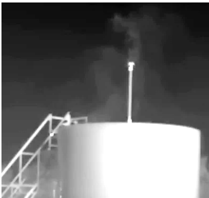
Intentional venting from storage tank
