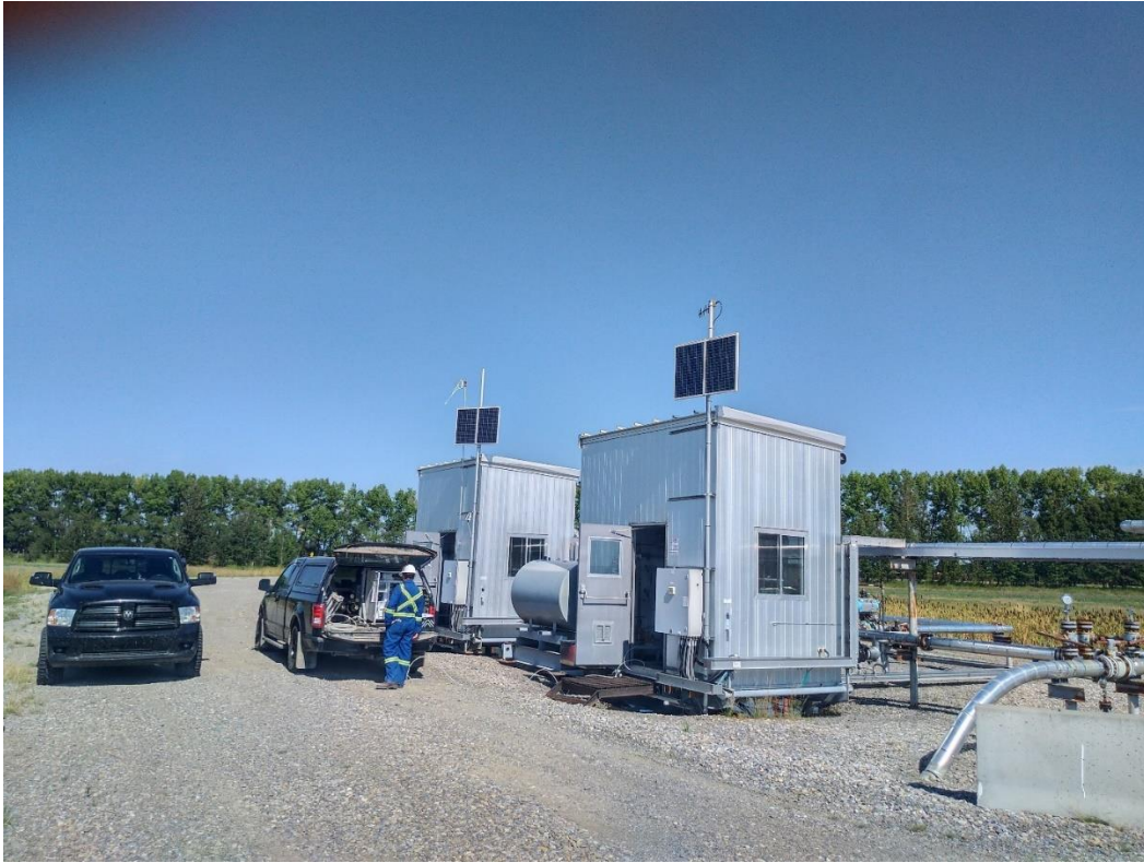
Picture 1. Photo of GreenPath and PTW at a double well battery in the Olds Field, measuring the vent rate of an optimized Bruin 5100 with a 1/2" plunger.
