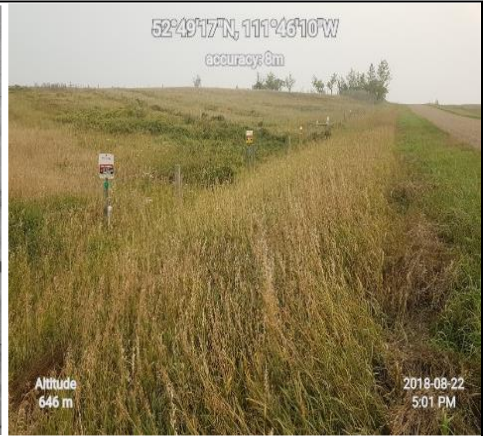
Photoplate: View south of start point of Segment 2A at KP 136.6; Highway 131 on the right of the photograph (12U 448149E 5852679N).
