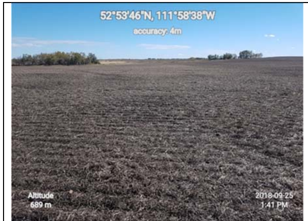
Plate D-7. View southeast across the abandoned pipeline segment near KP 120.8 at NW 21-45-14 W4M, also showing minor subsidence on the newer Line 3 to the right of the photograph.
