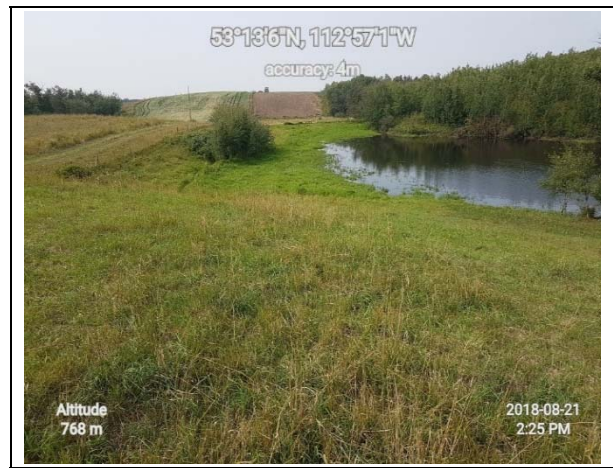
Plate D-6. View northwest across the abandoned pipeline segment showing a wetland to the east near KP 46.2 at NW 12-49-21 W4M.
