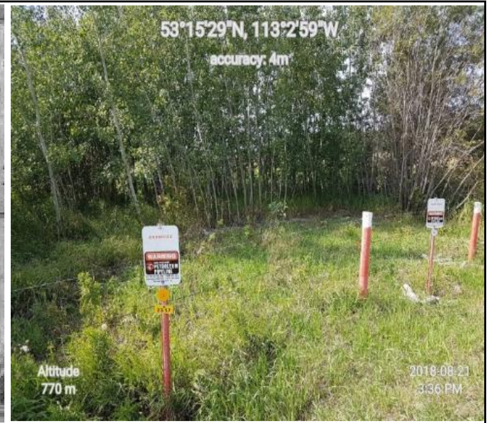
Photoplate: View northwest of abandoned pipeline segment showing tree regrowth adjacent to a road crossing near KP 38.2 at NE 30-49-22 W4M (12U 363272E 5902937N). This image was taken approximately 38 years after the abandonment of Segment 1A.
