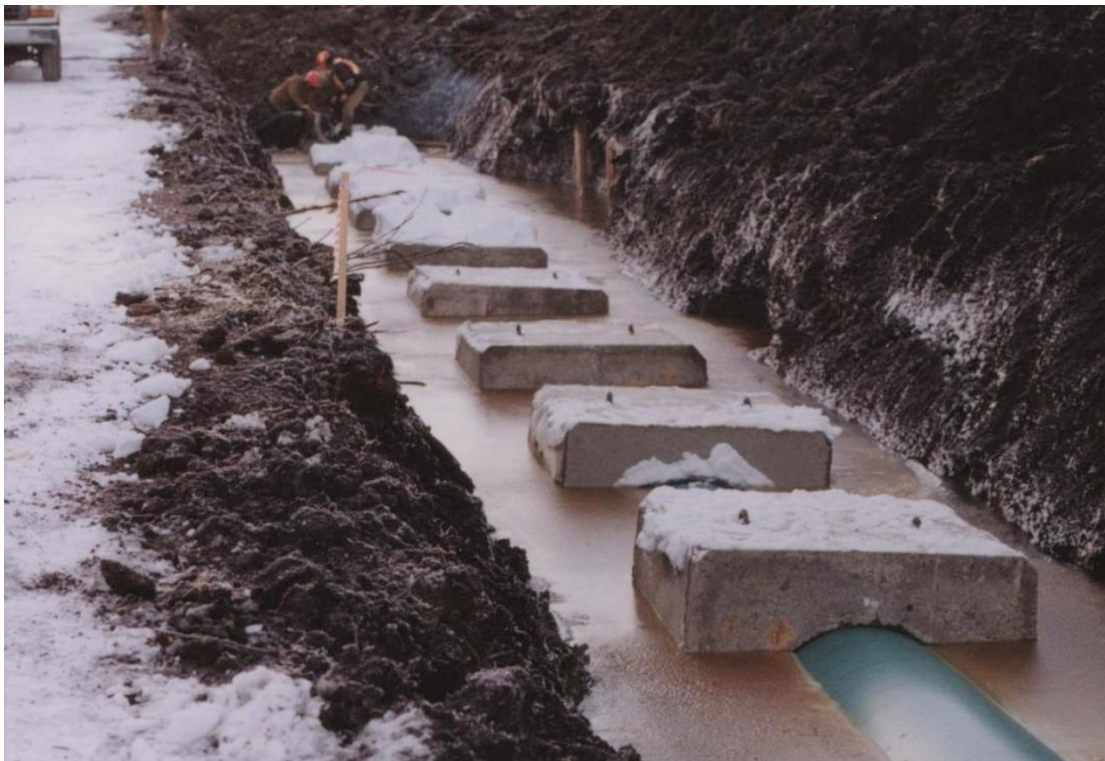
Figure 1 Concrete Saddle or Set-on or Swamp Weights (photo courtesy of T. Bossenberry)
