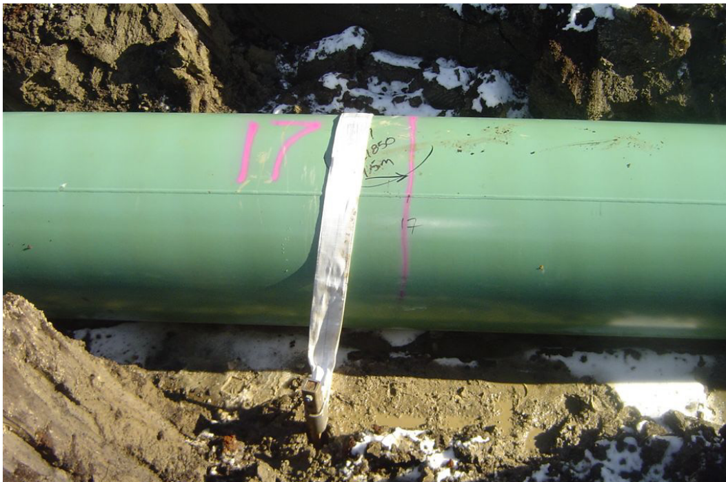
Figure 10 Example (2) Steel Screw Anchor and Polyester Strap Saddle and Connection (photo courtesy of A. Brown, AHB Consulting)
