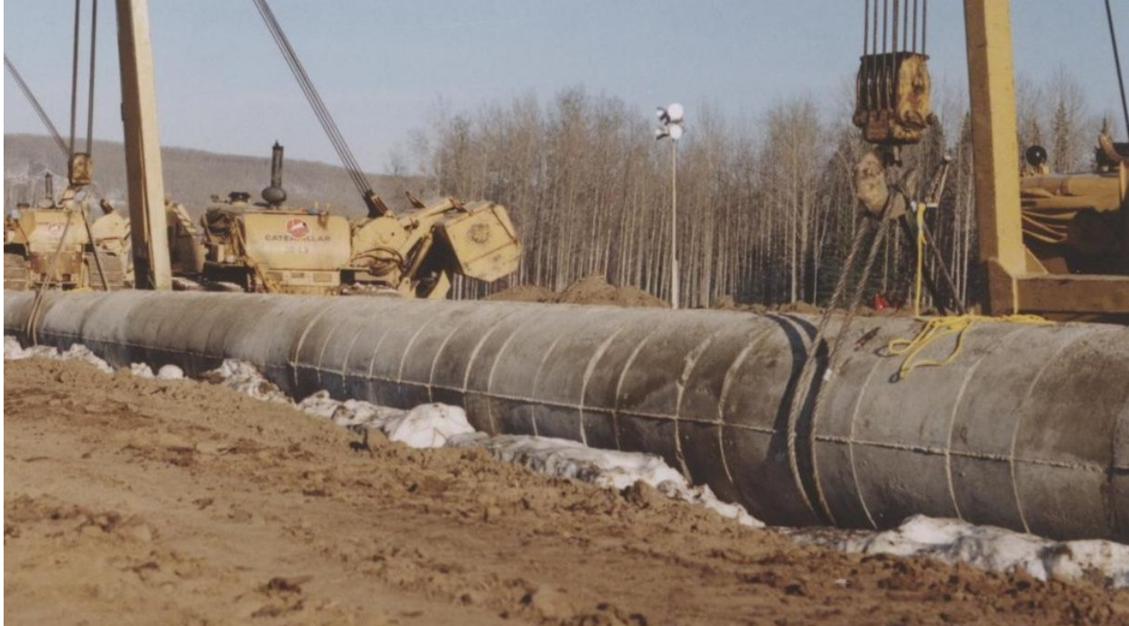
Figure 3 Continuous Concrete Coating (photo courtesy of T. Bossenberry)
