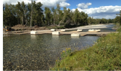
Simple temporary crossing.
