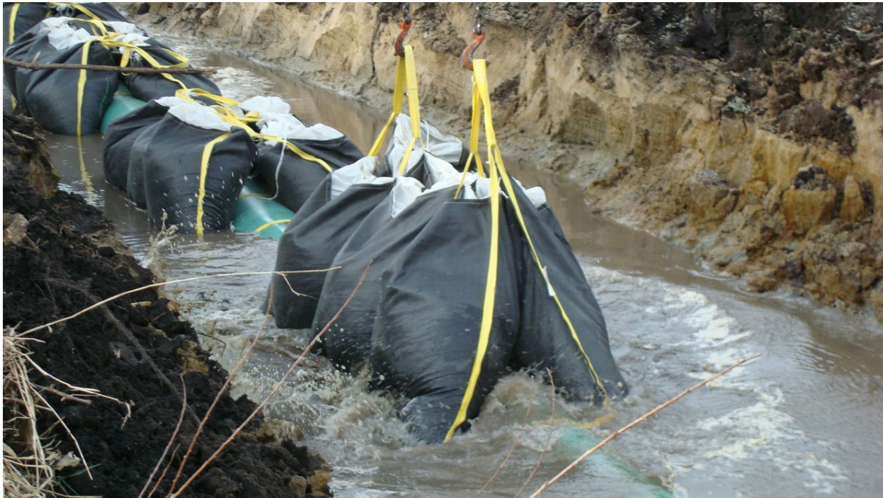
Figure 4 Soil (granular) Filled Bag Weights (photo courtesy of G. Connors, PipeSak®)
