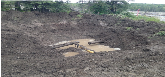
Bellhole excavation in bank or on a gravel bar.
