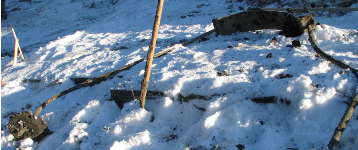
Figure 19 Excavated 40+ Year Old Screw Anchor in Northeast BC (photo courtesy of A. Brown of AHB Consulting)
