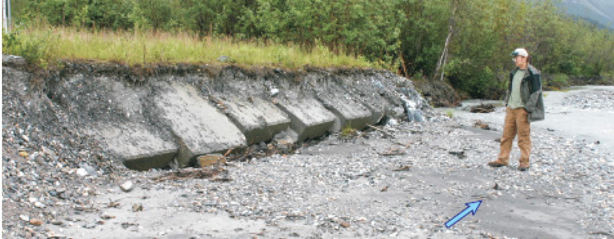
Figure 16 Saddle Weights Used as Bank Protection in Northern Alaska (photo courtesy of W. Veldman of WMV Consulting Inc.)
