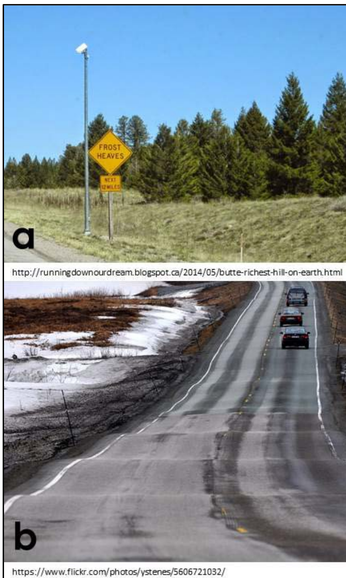
Figure B-1. Frost heave on roadways in a) Montana, USA, and b) Norway.
