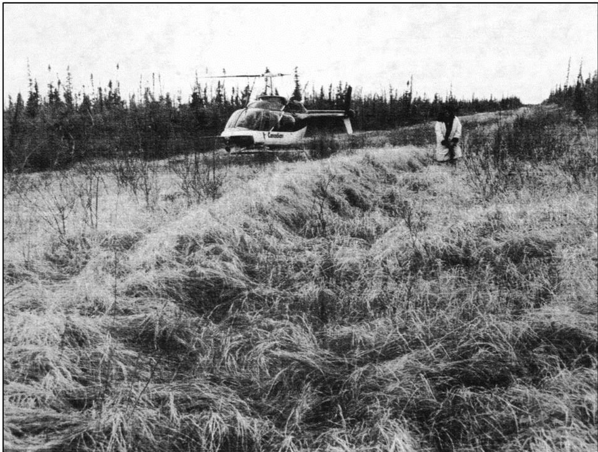
Figure 6.5: Upheaval buckling of onshore pipelines in Canada (after Nixon & Burgess, 1999).
