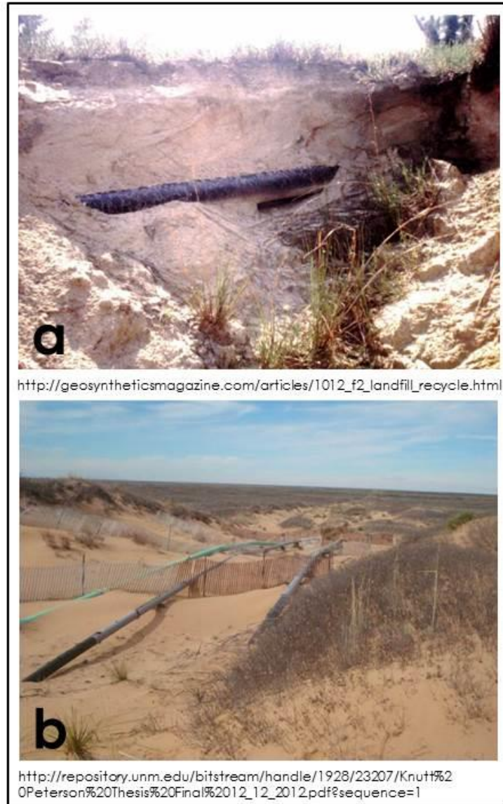
Figure 2.4: Soil degradation processes of a) water erosion or mass movement, and b) wind erosion, which have the potential to expose buried pipelines.
