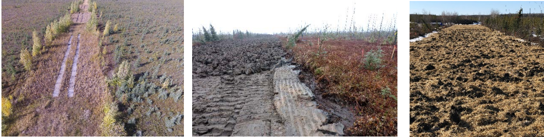
Figure 17. Partial Mineral Fill Removal – JACOS Road
